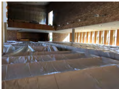
A sea of plastic protects the sanctuary during the roofing project.
